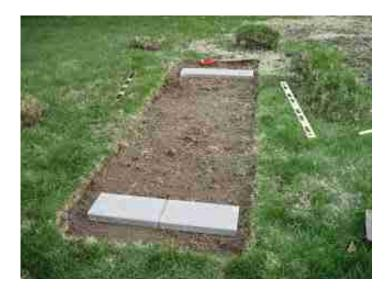
\*\*Although not shown, it is suggest to lay a weed barrier down before setting blocks and positioning rest of stand.
