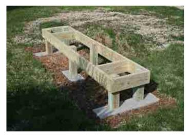
Getting the hives off of the ground is helpful in several ways. One, it provides better ventilation, and it also helps save your back when working the hives. And helps to keep some varmints out. This hive stand is built using treated lumber, and it should provide years of low maintenance service.
