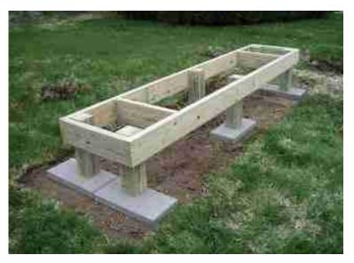
Here is the completed hive stand. It is 8' long, and 21" wide. This should support the bottom boards under the hives just fine. Added a stringer at each end for side support for the bottom boards. This should comfortably and safely hold 2 to 4 bee hives.
